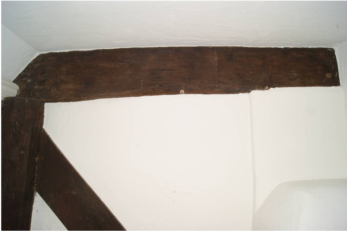
Figure 8 Sample location for OB06. Tiebeam south gable end. View south.
