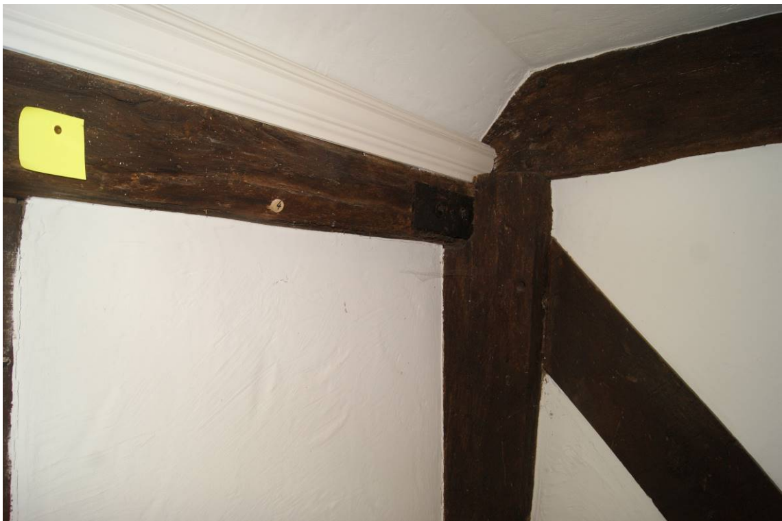
Figure 6 Sample location of OB04. Post west wall. View north west.
