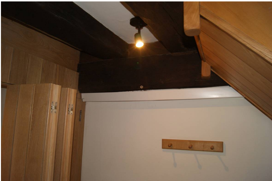
Figure 9 Sample location of OB07. Transverse beam in north gable. View north.
