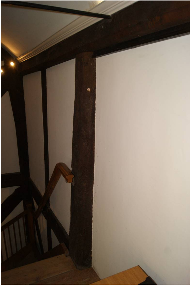
Figure 7 Sample location of OB05. Post east wall. View north east.
