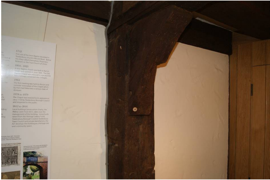
Figure 12 Sample location of OB10. Knee brace east wall. View east.
