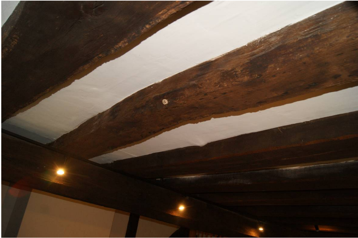
Figure 14 Sample location of OB12. Joist. View north.
